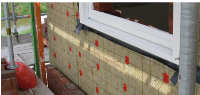
Prikspouwanker met UNI-CLIP
